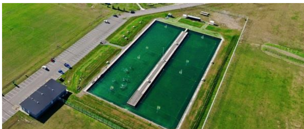
Figure 16 Hawke's Bay Canoe Polo facility.
