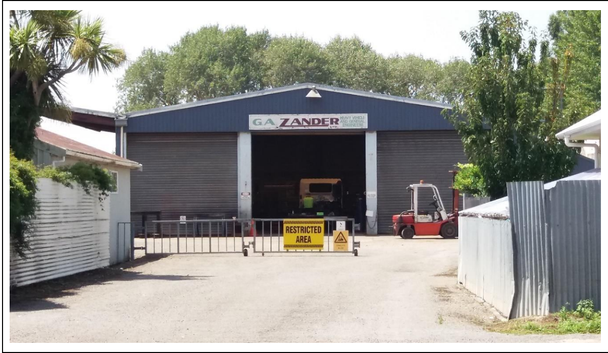
Photograph 4: General site condition, 573-575 Ruahine Street
