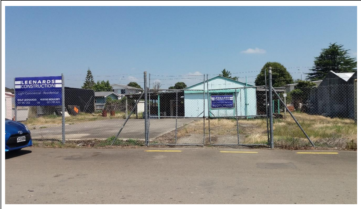
Photograph 2: General site condition, 29-31 Roxburgh Crescent
