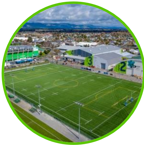
Redevelopment of the sportsfields at CETA
