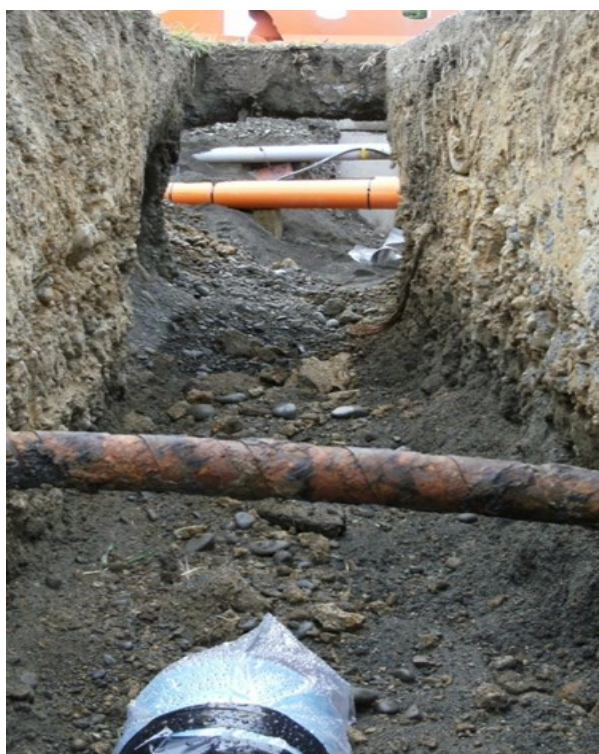
Figure A1 View from pipe end towards the duct
