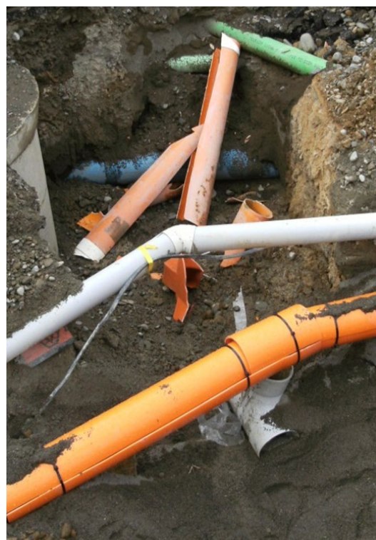
Figure A2 View of the repaired duct
