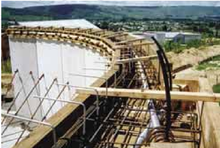
Construction of the second Ashhurst Reservoir, 1990.
