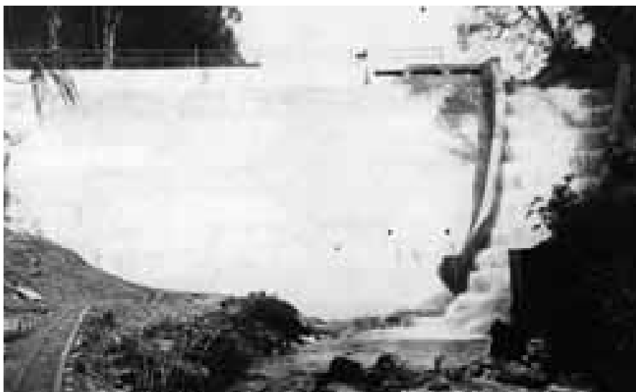
Opening Day 1913. In 1912, the second dam (built in 1907) was raised in height.
