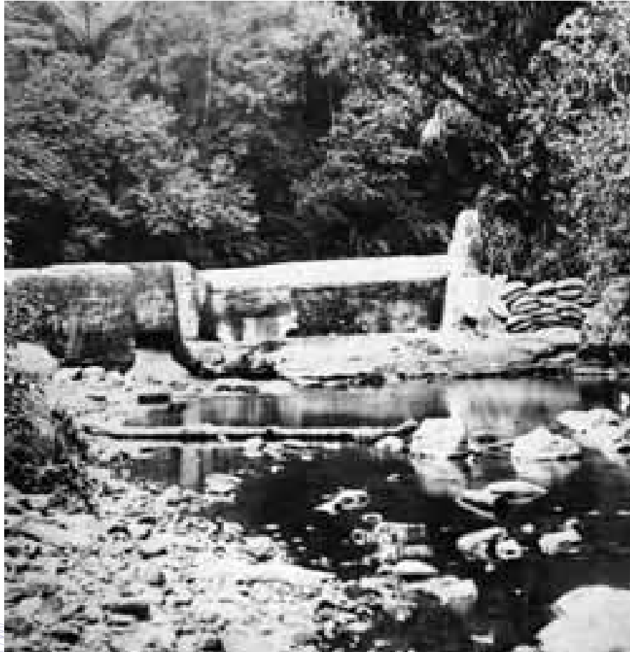
The original intake weir on the Turitea Stream, constructed in 1889.
