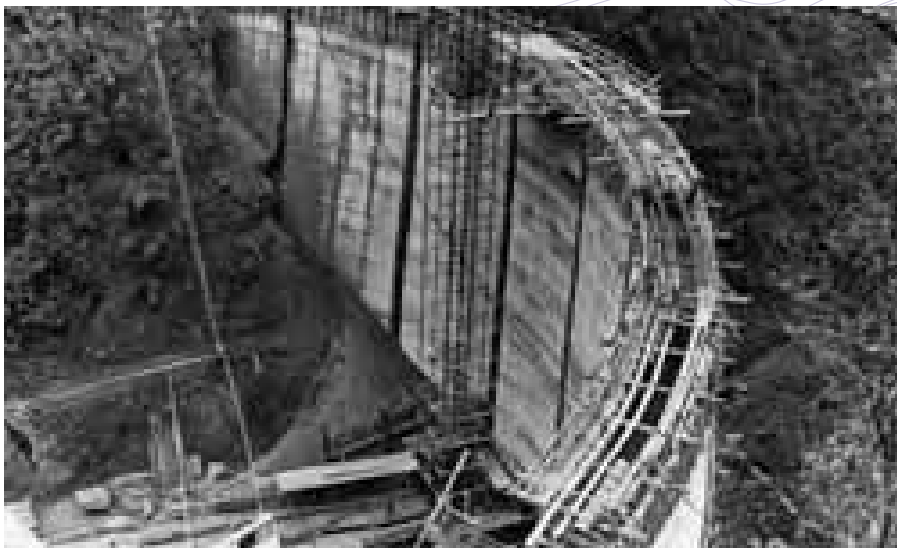
The upper dam progresses June 1955.
