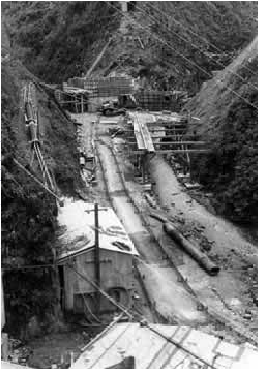
The upper dam under construction September 1954.
