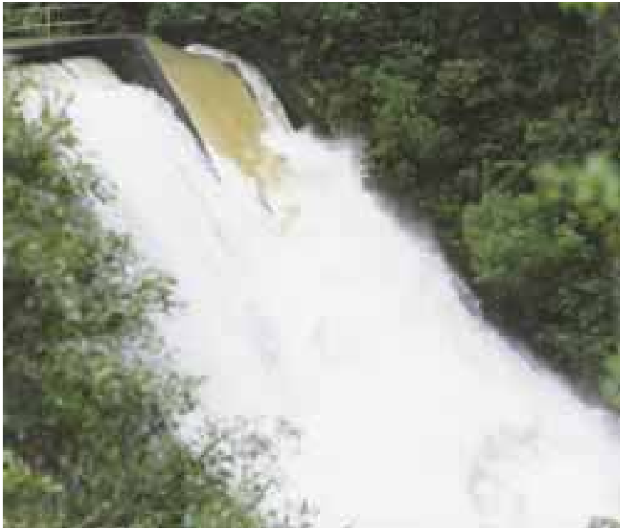
The lower dam in flood, August 1988.
