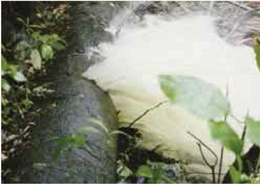
The original water treatment plant supply pipe gives up, January 1991.
