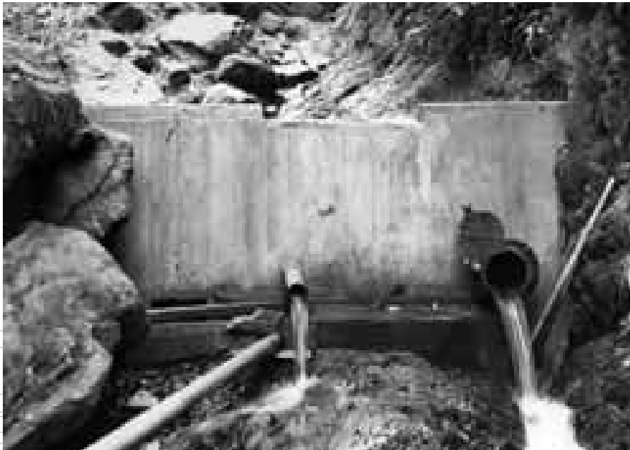
This weir was built in 1953 as an intake for pumping water to five 4500 litre tanks used for gravity water supply.
