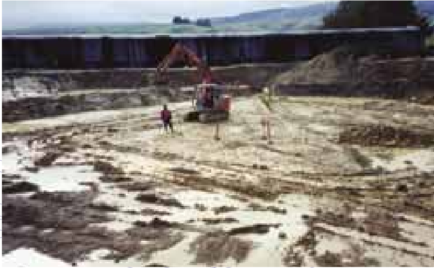
The construction of the second Ngahere Park Reservoir, 1998
