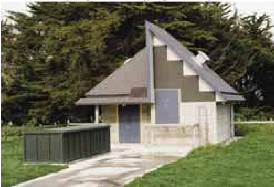
The Roberts Line bore pumping station. Photo circa 1990
