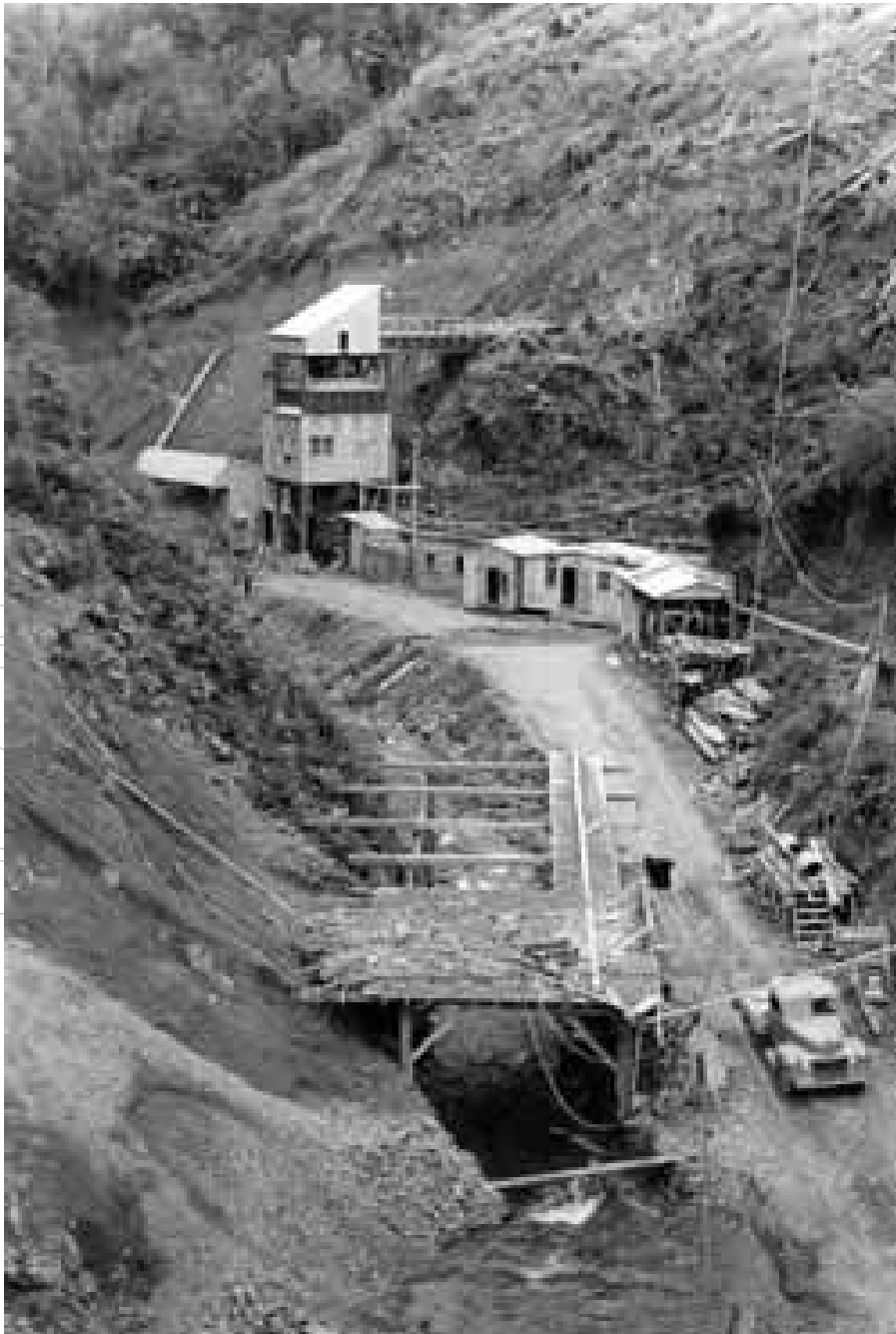
The batching plant and buildings, upper dam construction 1954.
