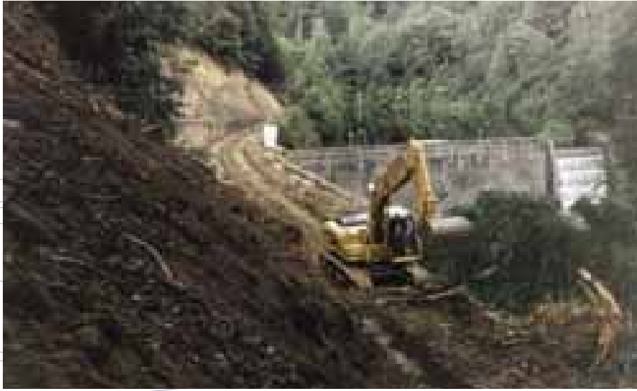
Beginning the second enlargement of the lower dam, May 1995.
