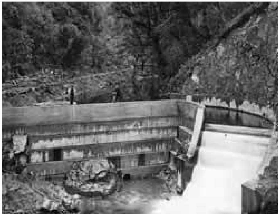
The Second Dam on the Turitea Stream in 1907. Samuel Jickell stands (on the left) atop his new dam. Note the fish ladder bywash.
