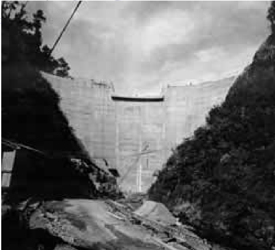
The upper dam nearing completion 1956.
