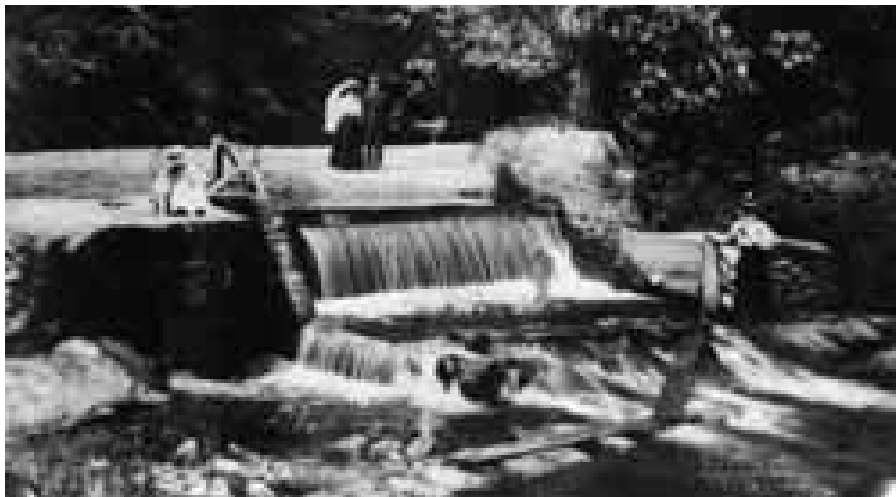
The original weir overflowing in 1911
