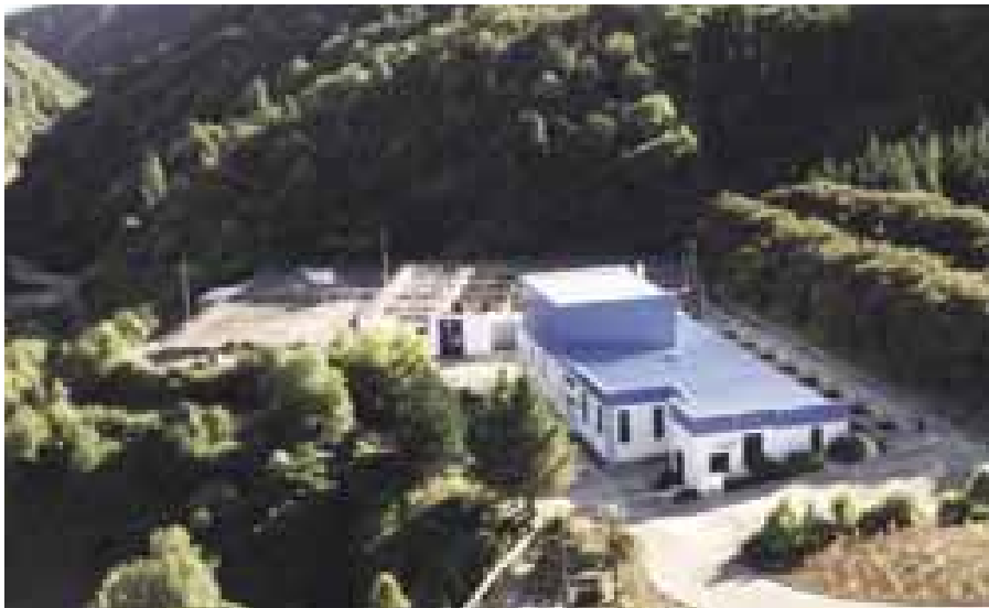
The Turitea water treatment plant after its upgrade in 1999.
